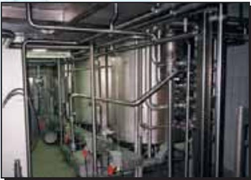
Leveltransmitters on CIP tanks
